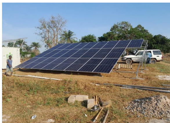
Partial view of one of the solar units being constructed
