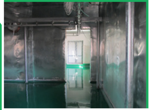
Construction process of cooling room at Arzni Meat Products slaughter house
