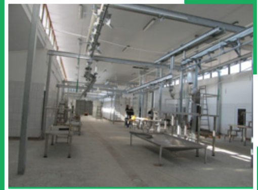
Installation of equipment at Zor LLC slaughter house
