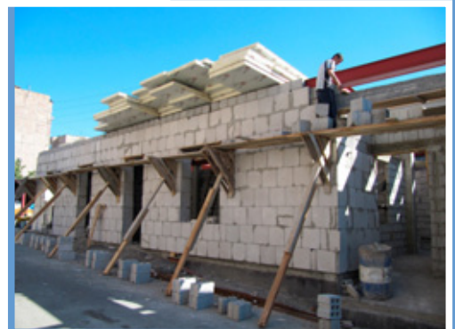
Pesticide Quality Control Laboratory construction site
