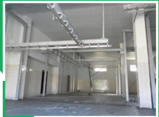
Installation of supporting railways at Khasik Titanyan's slaughter house
