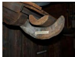
Rainwater gutter
