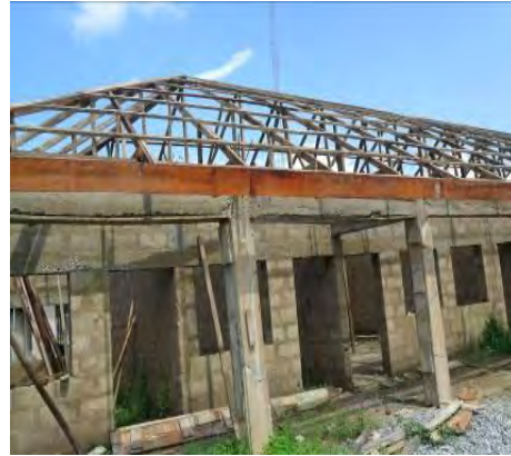
Plate 1b wood in the roof of a residential building
