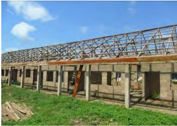
Plate 1 a: wood in roof of classroom construction
