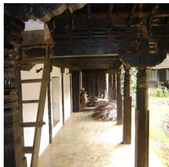
Figure 14 View of the wooden ceiling
