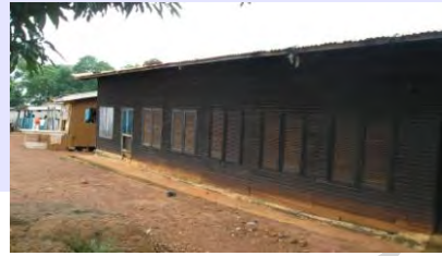
Timber house in a fair state
