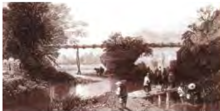
Figure 9: Bamboo water-pipe in Hongkong before 1983
