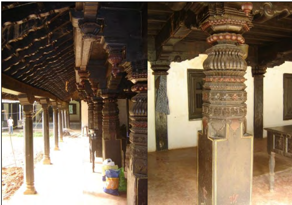
Ornamental Wooden Column and beams
