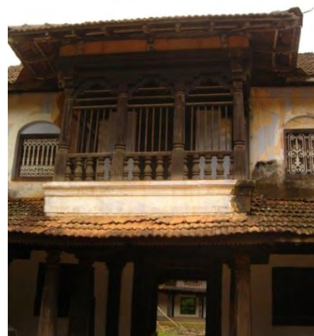
Figure 2: View of the balcony
