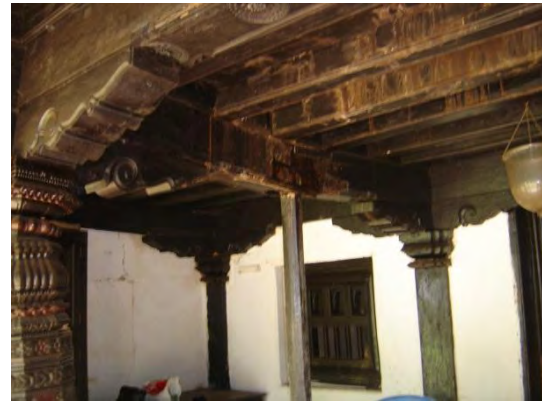
Figure 12: The treads are held by planks on either side
