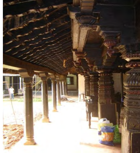
Figure 10: View of the heavy and the slender wooden columns
