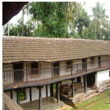
Figure 8 View of the corridor
