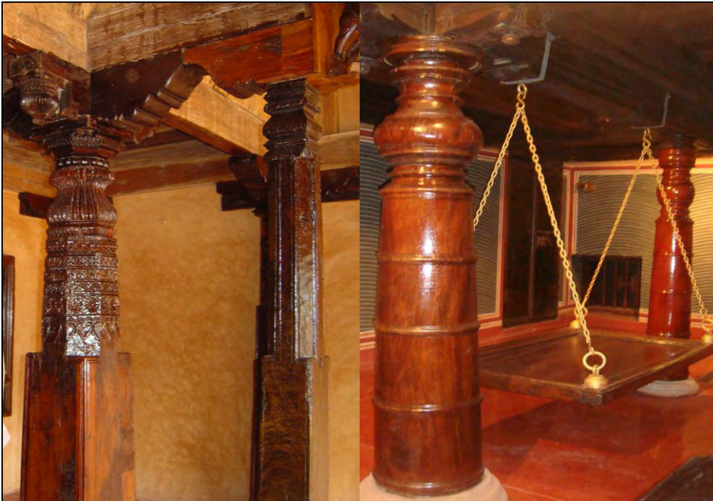
Ornamental Wooden Column
