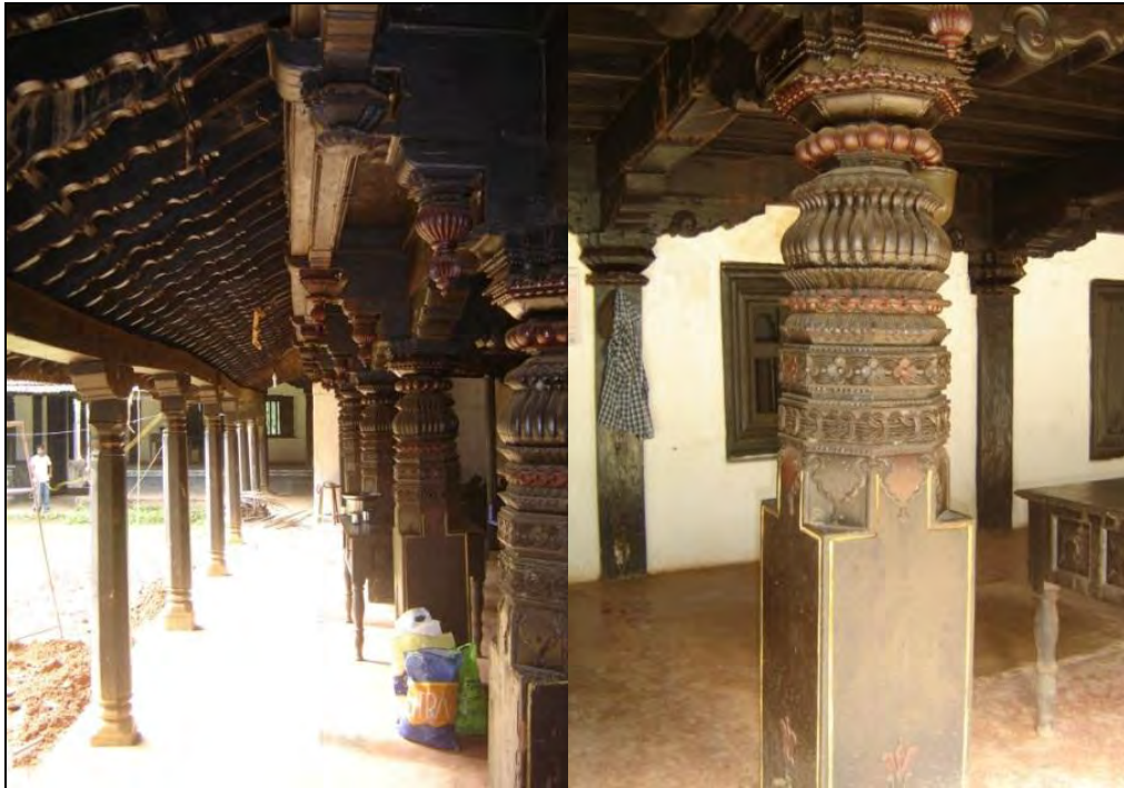
Ornamental Wooden Column and beams
