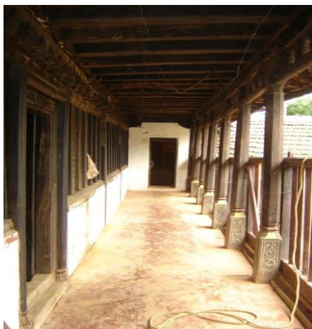
Figure 7 Slender columns in the corridor
