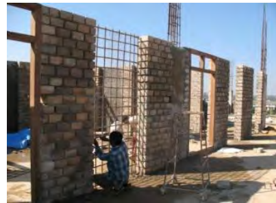
Figure 15: Bamboo Crete wall
