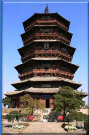
The oldest fully wooden pagoda in China - The Fugong Temple of Liao dynasty (1056AD). It reaches a total height of 67.31 m (220.83 ft).
