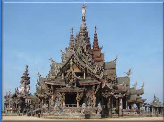
The Sanctuary of Truth in Thailand is a gigantic wooden construction. The top point of the building is about 105 meters high
