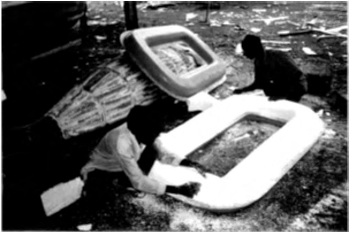
Fig. 15 Inserting polystyrene foam blocks into the half FRP shell of the prototype life float built in an FRP boatyard in Kakinada
