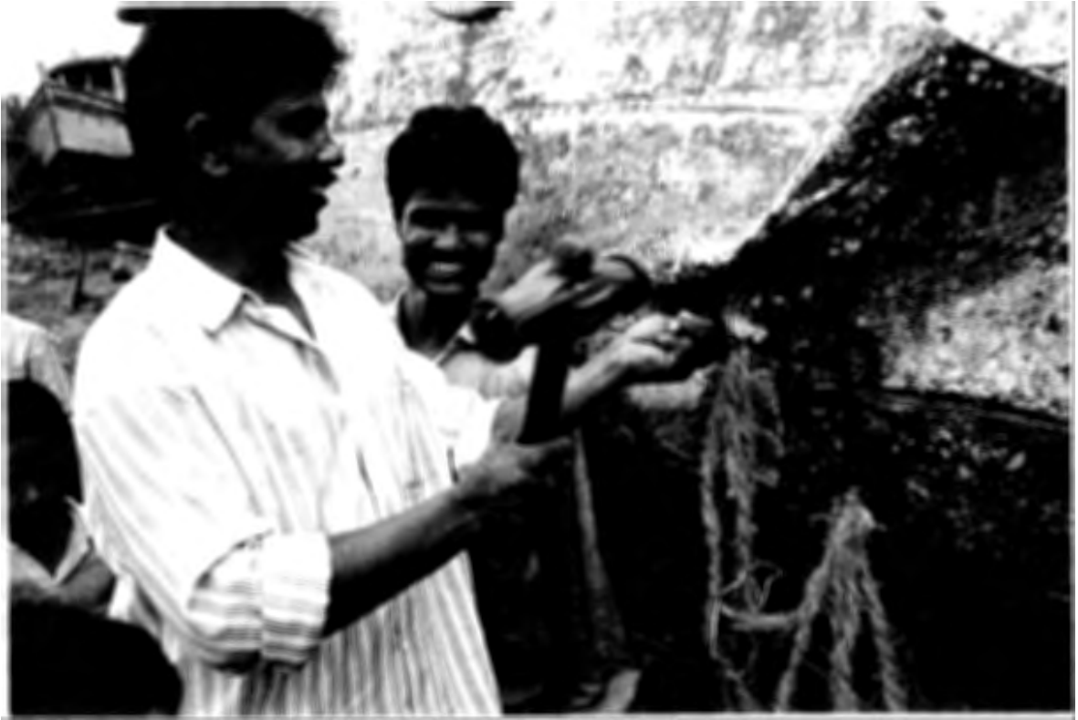
Fig. 10. A leak in a five year old trawler is stopped by massive caulking. The large gaps between the planks are caused by weak construction
