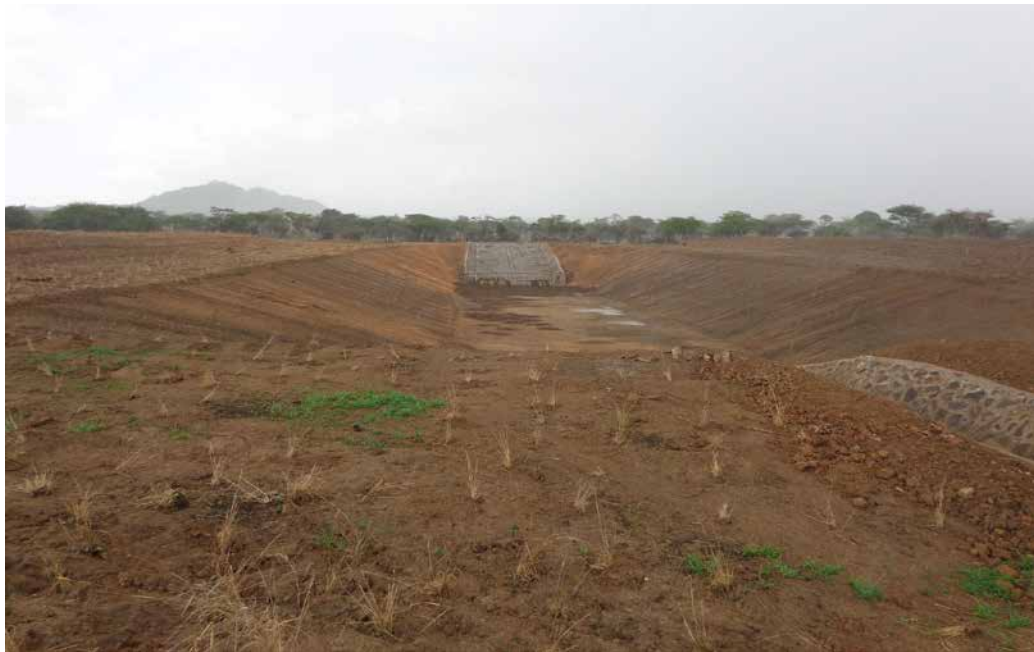
Figure 4: Excavated valley tank
