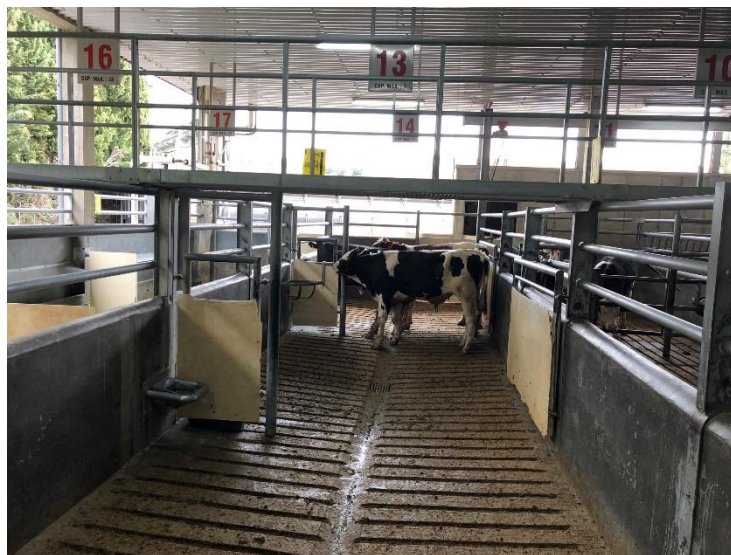
Figure 8. The lairage environment showing pen design and non-slippery flooring
