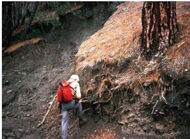
Figure 3.2 Ponderosa pine tree buttressing a slope above a forest road. Unprotected portion of road cut to the left has failed. Mendocino National Forest, California, 1978
