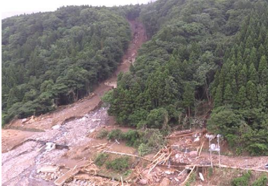
Fig. 5 Disruption of national roads due to runoff sediment (Kazama-ura village, Aomori Prefecture)
