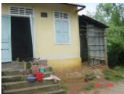
Ms. Gai's elevated, concrete house; the river is at the background.
