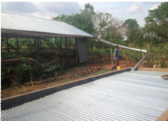
Figure 3. Rooftop rainwater harvesting with gutter and tank
