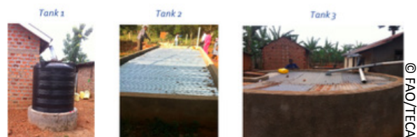
Figure 1. Different types of tanks for rainwater harvesting
