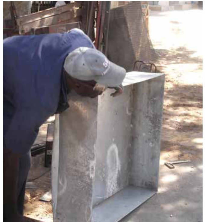
16 - Assembled metal box
