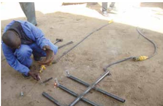
20 - Assembling the metal tubes that serve as air ventilation pipes
