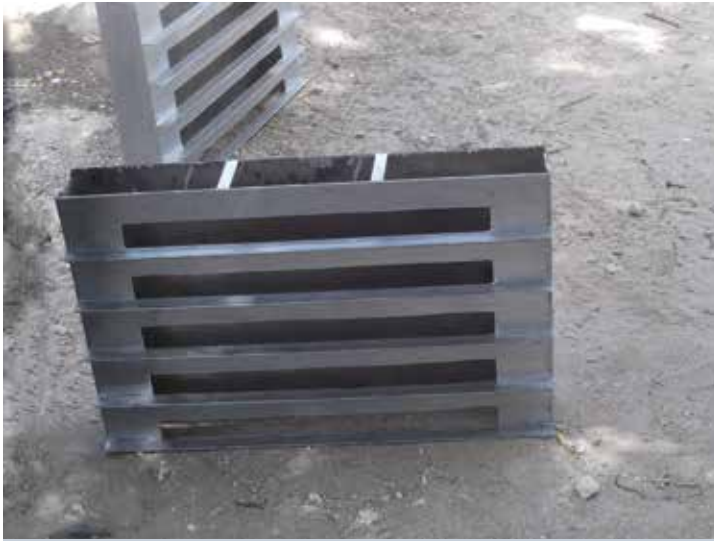
41 - Using a galvanized steel sheet to make the air outlet chambers
