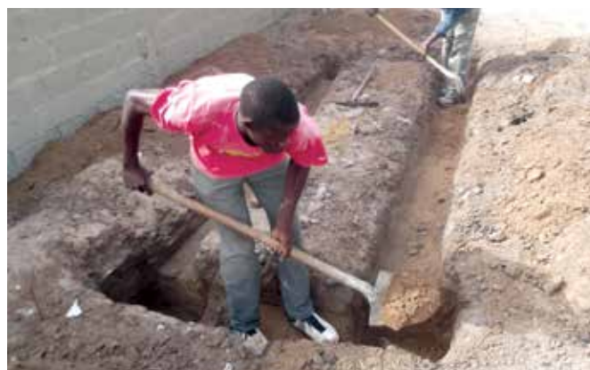
4 - Digging a 20 cm trench
