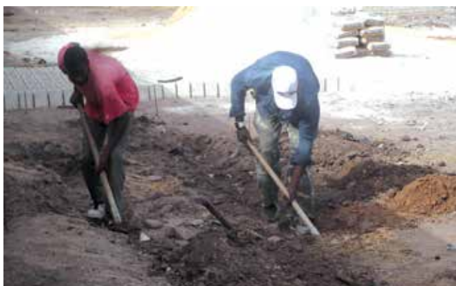
3 - Levelling the ground – foundation
