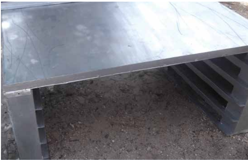
43 - Metal lid connecting the two chambers
