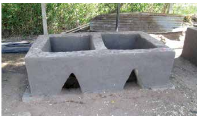
1 - Dual compartment frame (made with cement)
