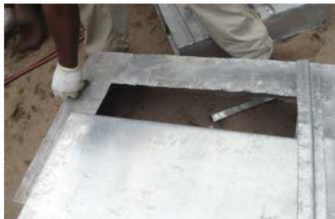
19 - Ash sheet inserted at the bottom of the box
