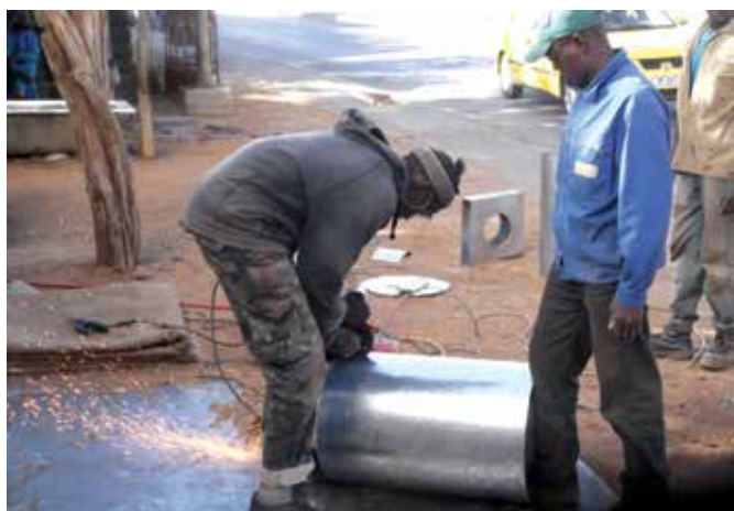
34 - Shaping the metal sheet into a cylinder to manufacture the barrel
