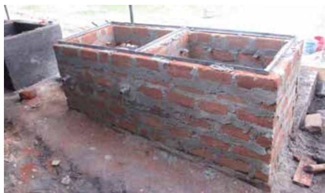
2 - Dual compartment frame (made with bricks)
