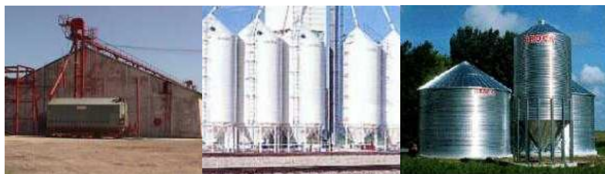
Figure 19. In bulk storage system, left: storehouse used mainly in developing countries, middle: concrete silos used in storage centres, right: corrugated-steel silos for on-farm storage.
