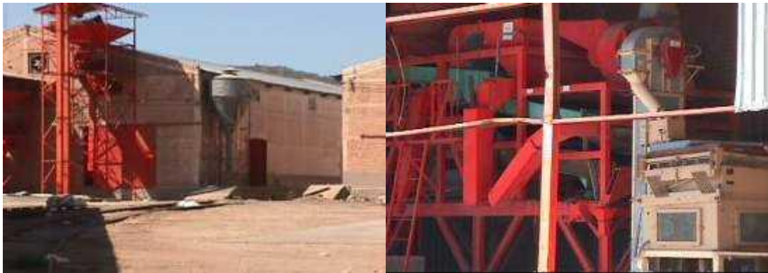
Figure 15. Grain cleaning equipment, left: overall view; right: close-up.
