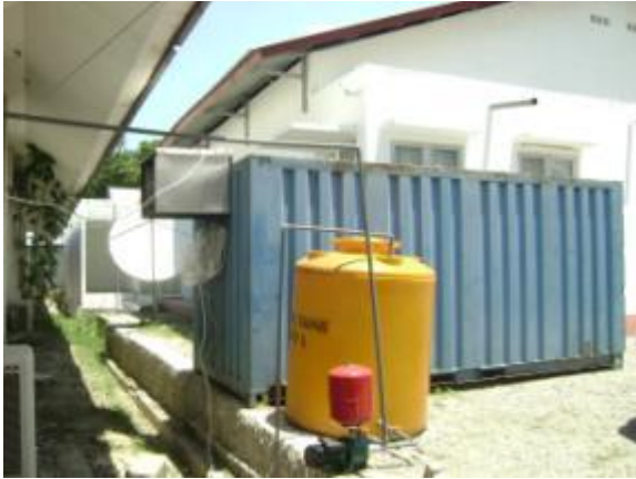
The dedicated storage container in the background. In the foreground is the water pressure pump, which serves as the water supply line for the automated ice machine.
