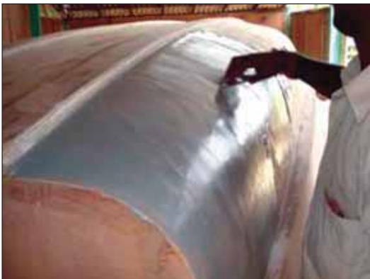
Figure 51 Applying autograde putty.
