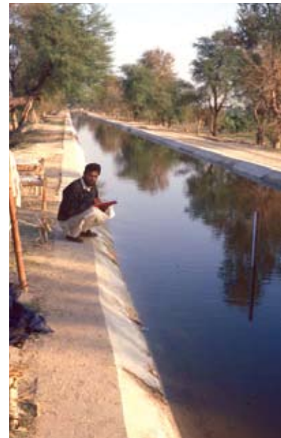
Measurement of seepage losses in Fordwah-Sadiqia, Punjab, Pakistan.
