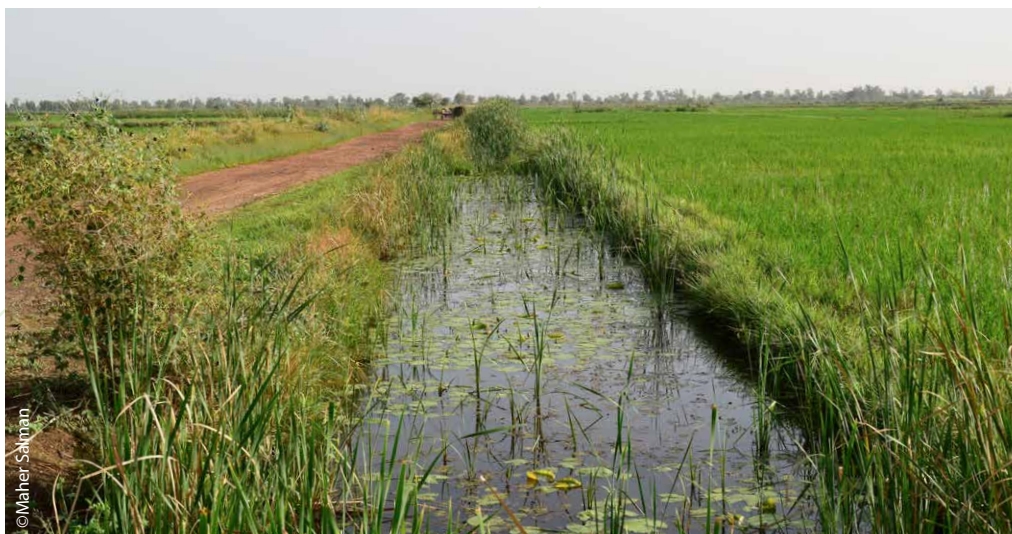
Figure 12: Main drain network in Ben Nafa Kacha, Burkina Faso
