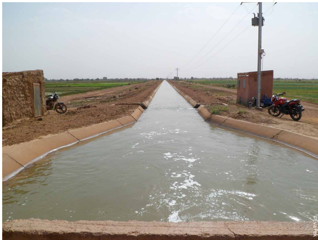
Figure 10: Main canal of Ben Nafa Kacha, Burkina Faso
