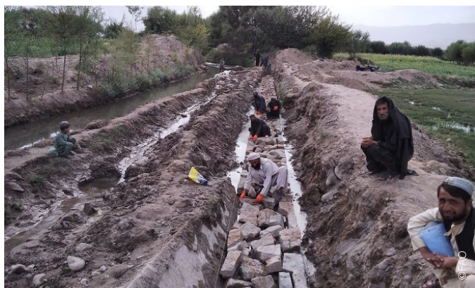
Rehabilitation of 50 meter water canal for irrigation.
