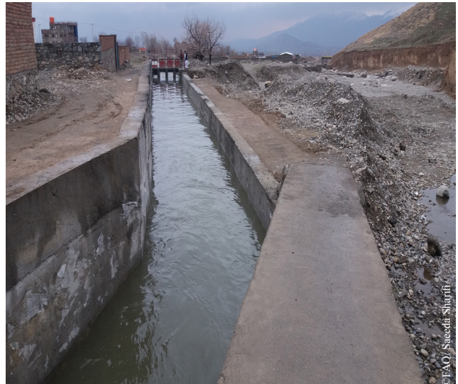
Sediment Trap for Feeder Canal of Qargha Dam
