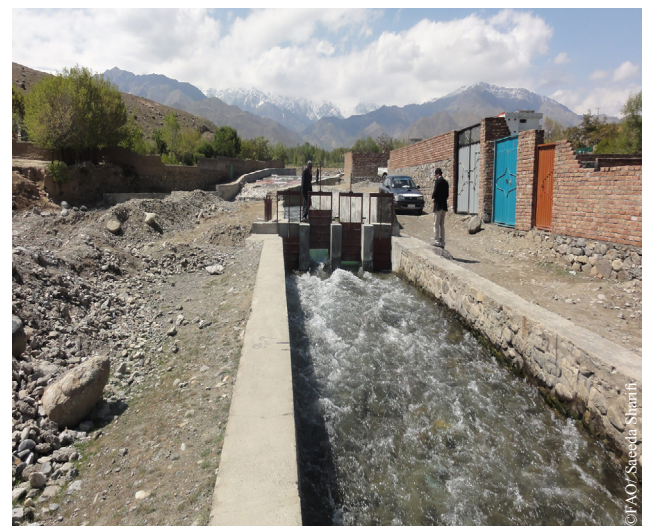
Regulator of Qargha Dam Feeder Canal
