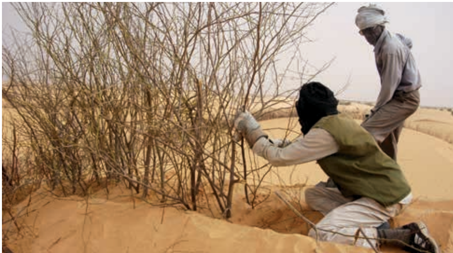
Installing a palisade, mechanical dune stabilization, Mauritania
