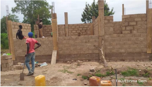
Ongoing construction of school kitchen with improved cooking stoves
