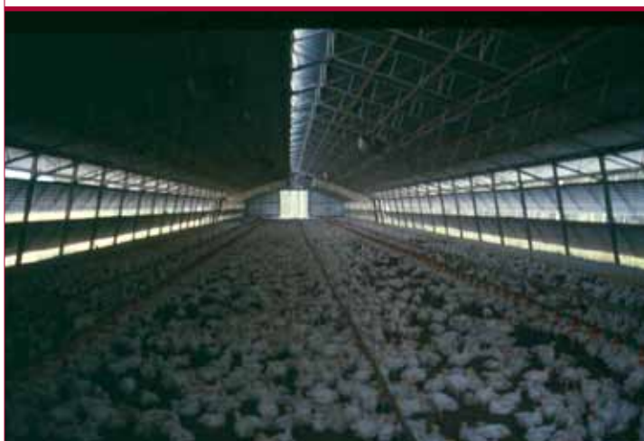
Large-scale naturally ventilated broiler house
