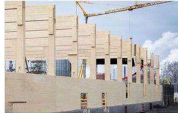
Cross-laminated timber – CLT
