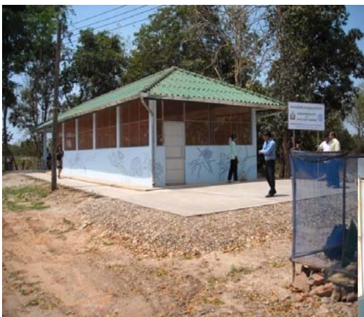
Demonstration site – outside view
