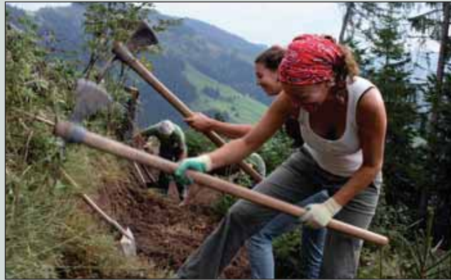
Construction of access trails, Entlebuch, Switzerland
