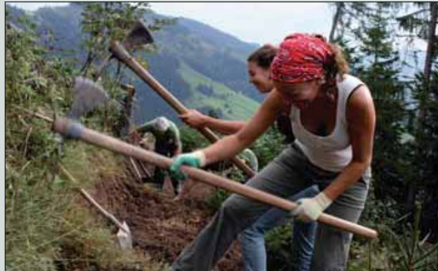
Construction of access trails, Entlebuch, Switzerland
