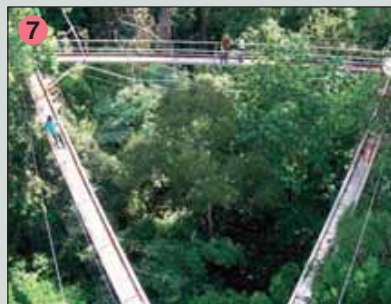
This aluminium alloy canopy walkway in Pasog, Malaysia was constructed in 1992 as a collaborative project between the Forest Research Institute of Malaysia and Japan's National Institute of Environmental Sciences
