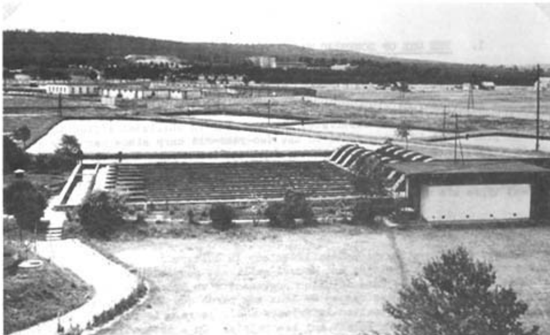
Fig. 1 Kielce sewage treatment plant and fish ponds. Photo: P. Wolny
