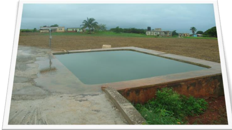
Concrete catchment and reservoirs with solar driven submersible pump Location: St. Elizabeth
