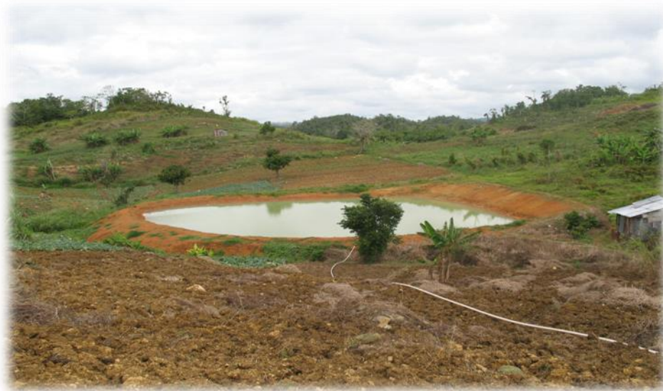
Figure 21: Excavation pond with no sealing
