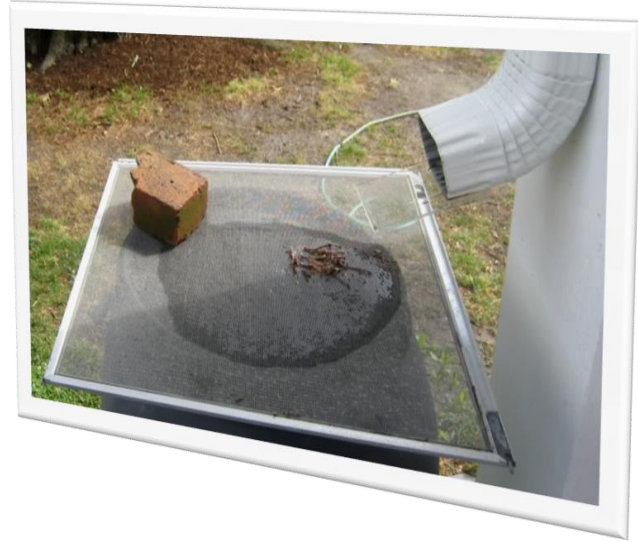
Downpipe and storage barrel with a simple screen
