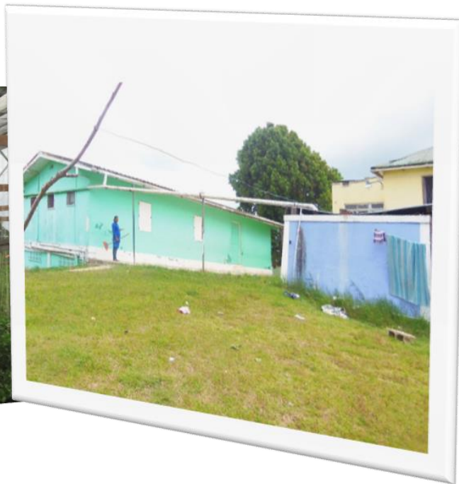
Rainwater harvest system for school operations
