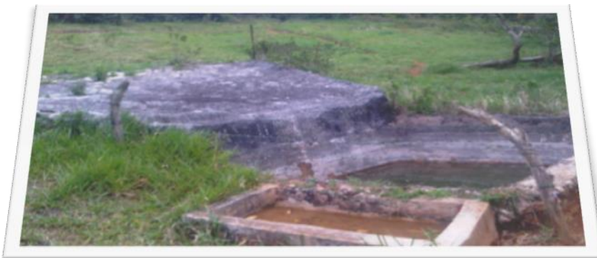
Rain water harvest system for livestock - Manchester, Jamaica
