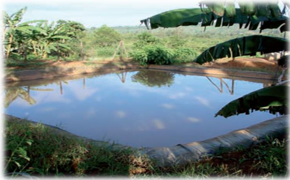
Figure 19: Lined reservoir in Manchester, Jamaica
