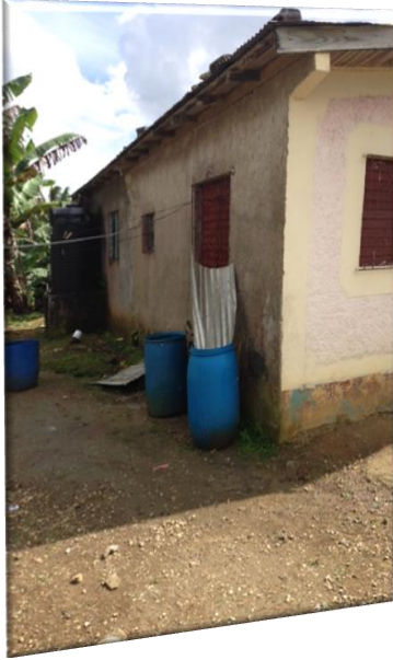
Simple system with barrel and zinc
