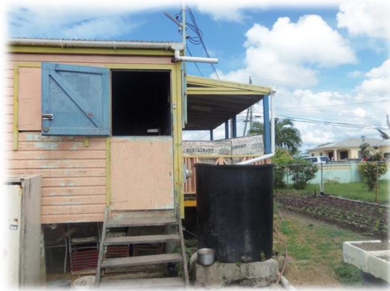
Figure 30: Rainwater harvest system for backyard gardening in Antigua
