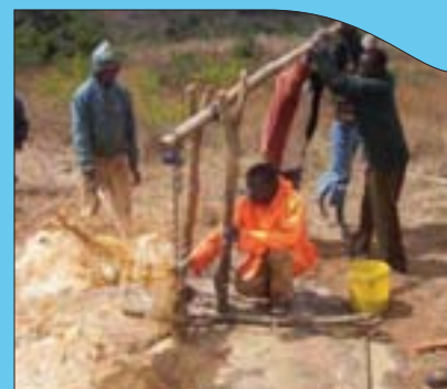
FIGURE 4. Training of drilling team in rota sludge technology for well development – Practica Foundation
