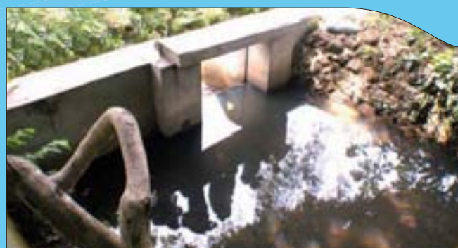
FIGURE 33. Diversion weir & Intake structure in Wetland Development - SPFS Guinea
