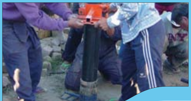
FIGURE 6. Installation of tubewell with locally adapted materials – SPFS in Madagascar
