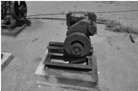
Picture 1: Borehole with pump
