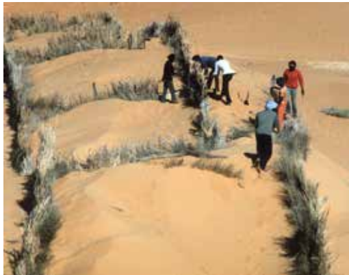
1990- FAO Dune Fixation and Stabilization Project helped fight against desertification in Mauritania, especially where sand dunes encroach upon agricultural land.
