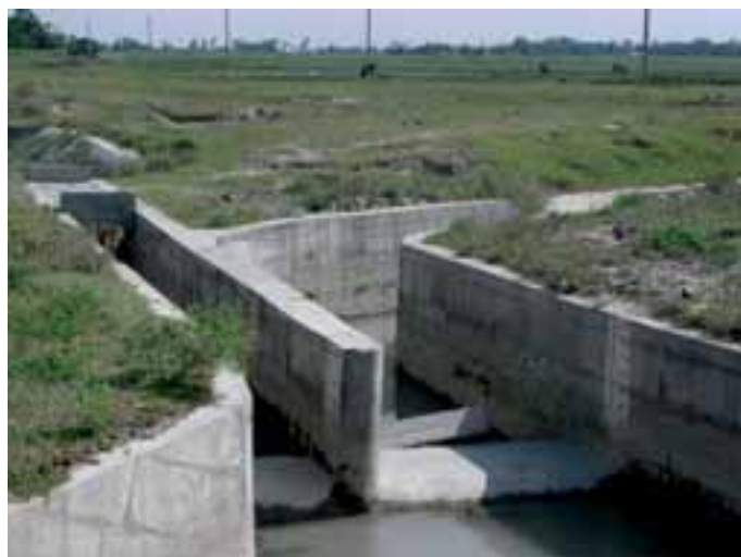
Plate 1 Proportional fixed divider structure seen from upstream, SMIS, Nepal.
