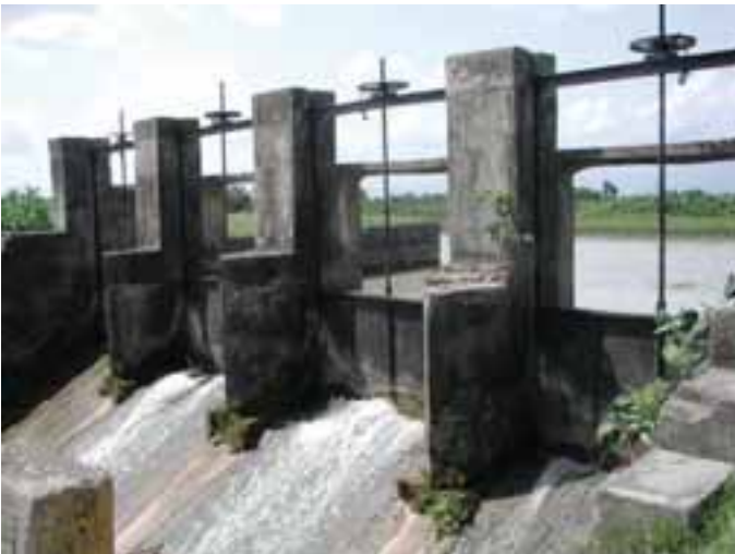
Plate 3 Side-gated structure (escape), SMIS, Nepal.
