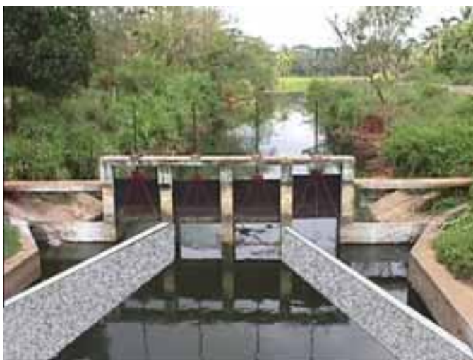
Plate 31 Building side weirs on gated regulators.
