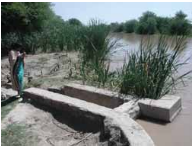
Plate 26 Uncontrolled direct outlets on the main canal as sources of perturbations, Sindh, Pakistan.
