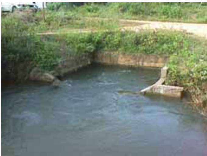
Plate 16 Offtake with downstream submerged conditions.
