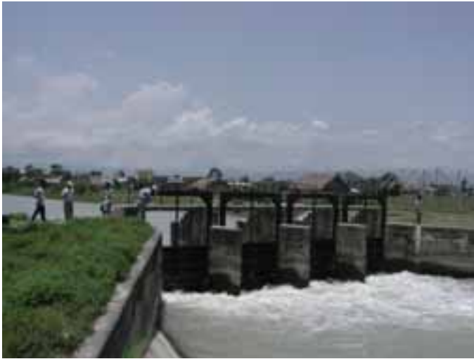
Plate 2 Slide gated cross-regulators, SMIS, Nepal.
