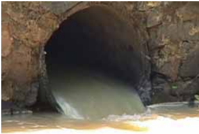
Plate 17 Offtake with free-flow downstream conditions.
