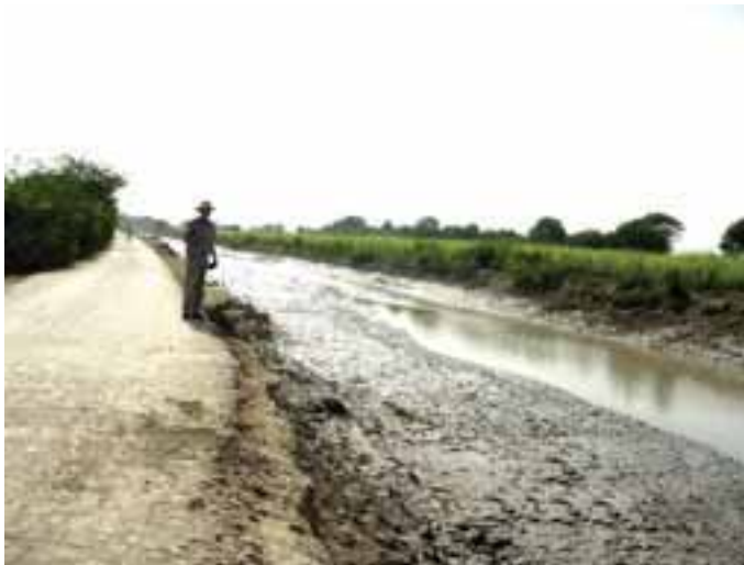
Plate 15 Reduced carrying capacity of a canal because of sedimentation, Fuleli, Pakistan.
