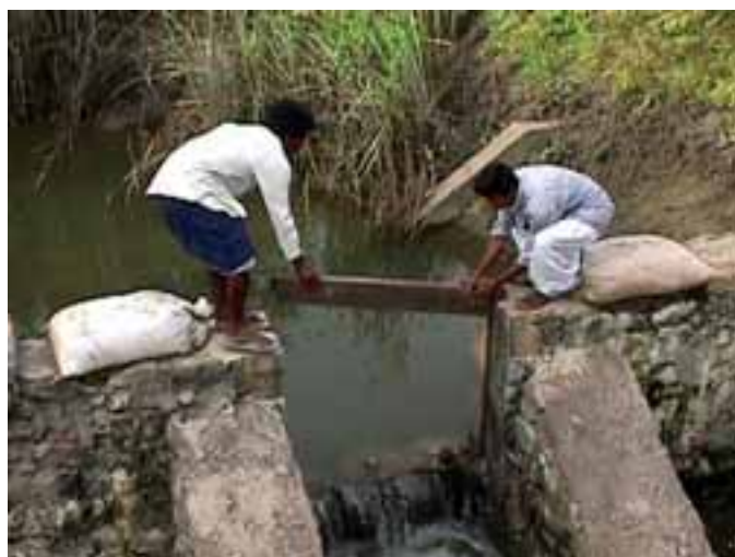
Plate 8 A step-by-step regulator, Sri Lanka.
