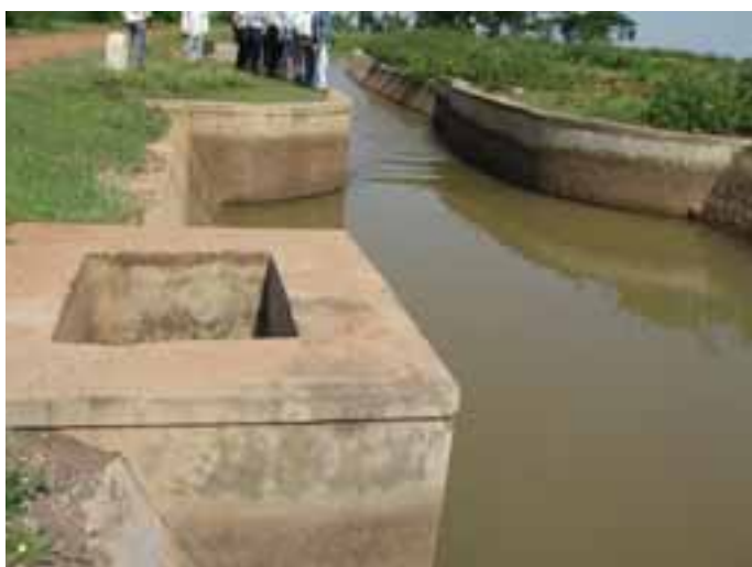
Plate 20 Measurement capacity: submerged flume with no critical section, yielding incorrect measurements GLBC, Karnataka, India.
