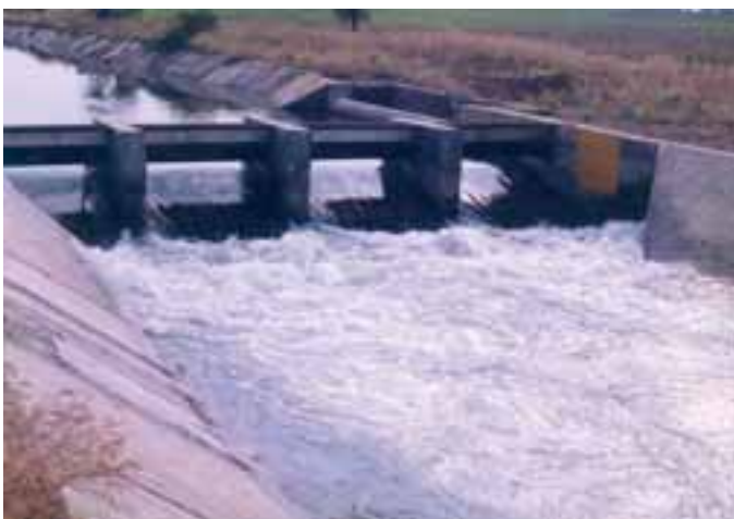
Plate 4 Fixed side-weir with cross-deflector, Maharashtra, India.
