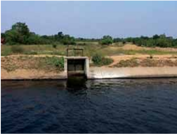
Plate 7 Diversion control structure (offtake).
