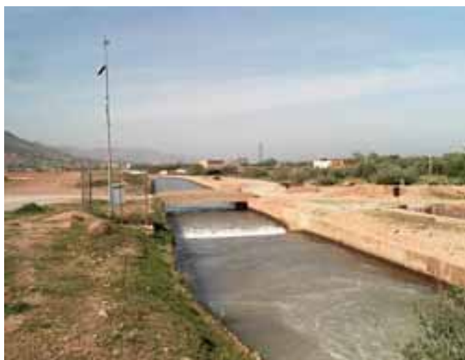
Plate 5 A measurement station with remote terminal unit, Morocco.
