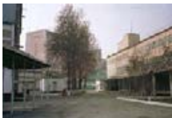
The second milling facility (to the right)
