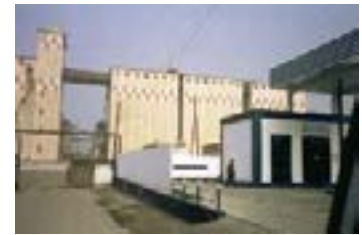
The 50,000 t elevator
