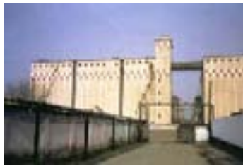
The 50,000 t elevator
