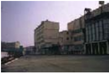
The major mill connected to the elevator
