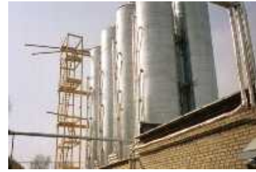
Malt storage facility
