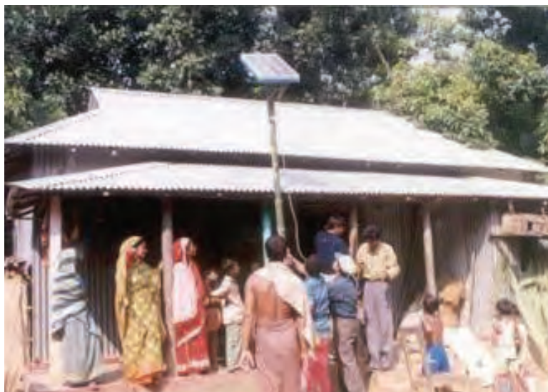
Plate 2. Installing a solar panel
