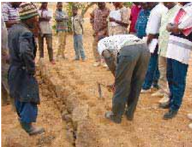
Communal stone rows laying.
