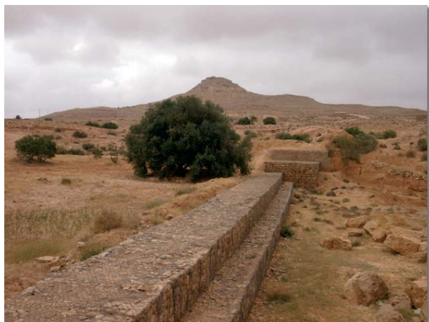
Dry stone walls are among the many practices developed to prevent soil erosion
