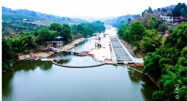
A fish passage was built at the Xiaojiatan Barrage in Jiangjin in April 2022.
