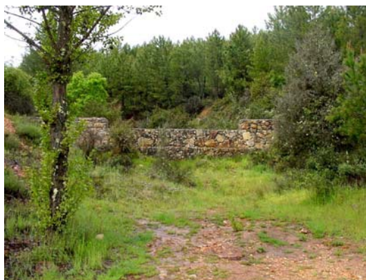
Fig 3. Gavion masonry stabilisation dam.
