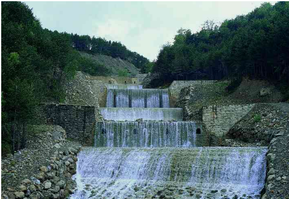
Photo 5: Correction work achieved in the last years (picture from 2001)
