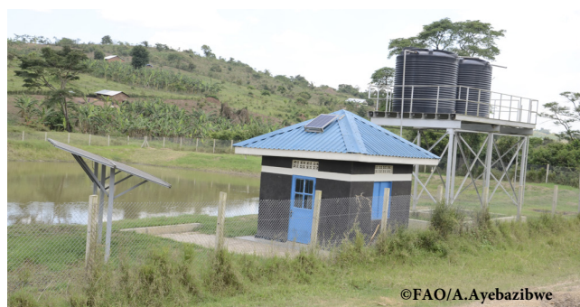
One of the valley dams constructed under FAO's Global Climate Change project funded by the European Union, in Mubende District
