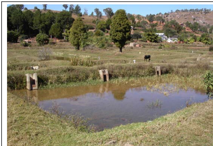
Figure 1: Abandoned and semi-abandoned government fish stations can be found in nearly all countries. Unless divested, they pose a drain on public coffers, a poor use of resources and sometimes a public health risk (Madagascar).
