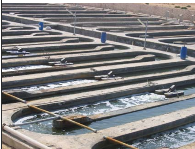
FIGURE 8 D-ended shape tilapia raceway (145 m 3 ) with 2 HP air-injector, in Valley Organic company, El-Beheira Governorate, Egypt
