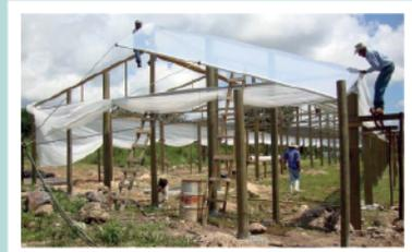
Figure 1. Installation of covering materials for a low-cost greenhouse
