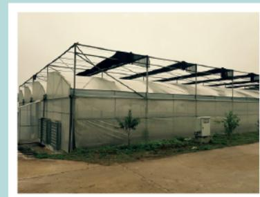
Figure 11. An expanding/retracting net system for efficient management of shade
