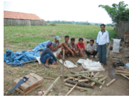
Building new cages at destocked layer farm in Indonesia. Photo: Ian Douglas
