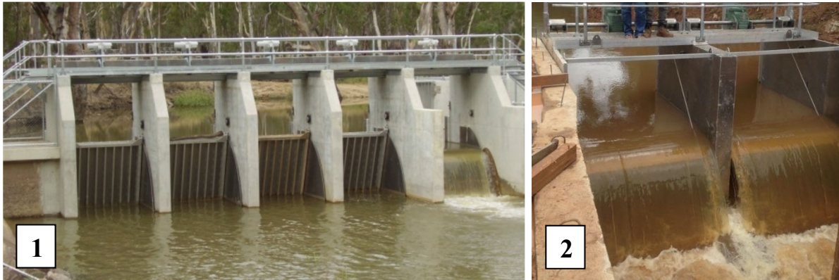
Figure 13: (Left) Best practice regulator from the Yallakool Creek, Australia. An ageing, leaky, undershot regulator was replaced with a tilting overfall design, which contained a deep plunge pool so that fish did not hit the abutment when moving downstream. The regulator now also includes a fish ladder so fish can move upstream. (Right) Best practice regulator from Pak Peung wetland, Lao PDR. This overfall regulator is also constructed together with a plunge pool. It too is associated with a fishway (Figure 10 above). (Photo credit: 1. AWMA Pty. Ltd. Australia; 2. Lee Baumgartner)
