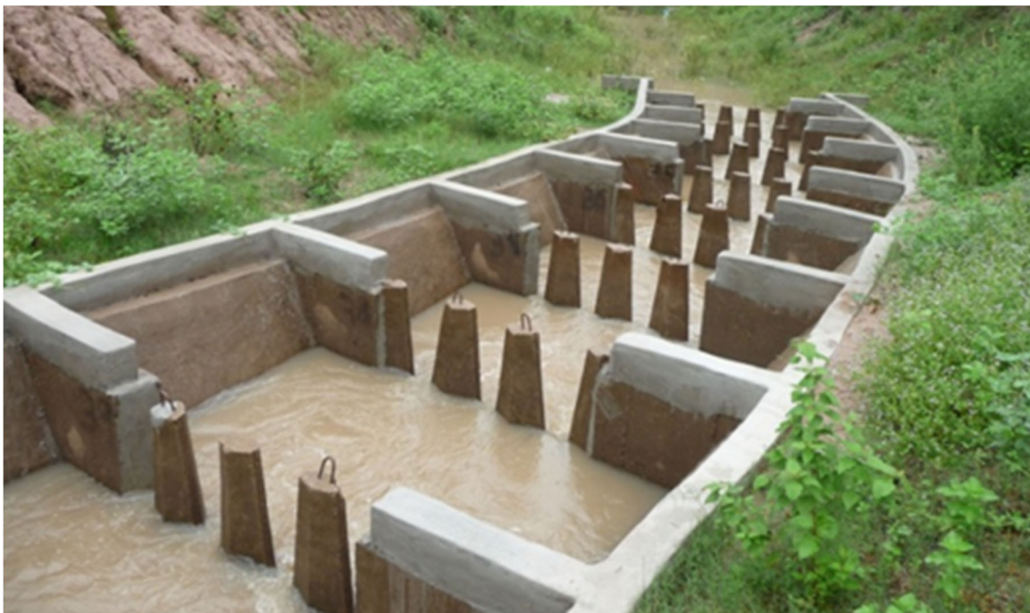
Figure 10: Example of the “cone-type” Pak Peung fishway (Lao PDR), in a tropical irrigation system. (Photo credit: Lee Baumgartner)
