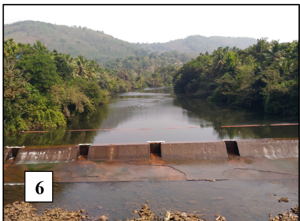
Figure 6: Examples of common irrigation structures and other associated structures, which obstruct fish passage. (Photo credit: 1. Sukanvk2000; 2. Rick Gregory; 3. Lee Baumgartner; 4. Rick Gregory; 5. Vinayaraj V R; 6. Vijayan Rajapuram)
