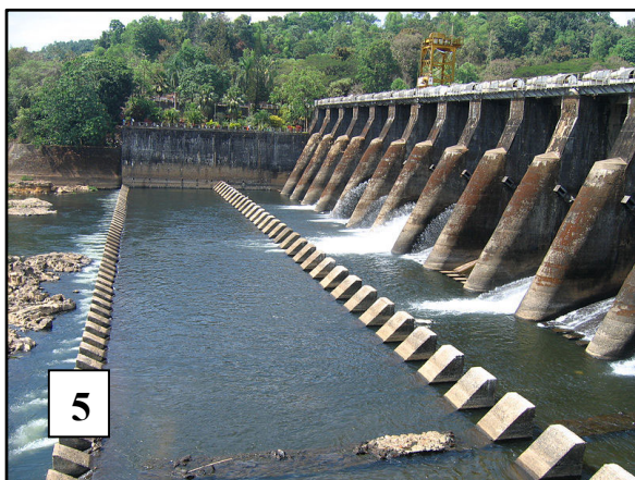
Figure 6: Examples of common irrigation structures and other associated structures, which obstruct fish passage. (Photo credit: 1. Sukanvk2000; 2. Rick Gregory; 3. Lee Baumgartner; 4. Rick Gregory; 5. Vinayaraj V R; 6. Vijayan Rajapuram)
