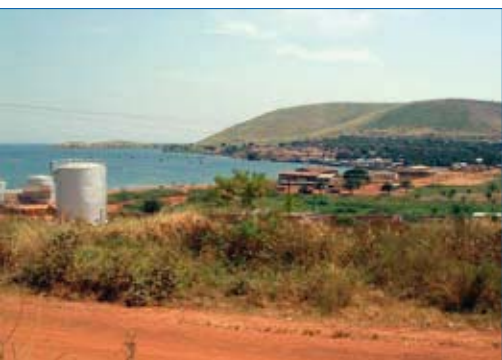
Kigoma Harbour, oil storage tanks
